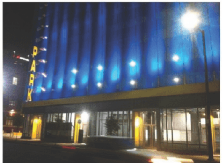
*ACTUAL PICTURE OF PARKING GARAGE*
